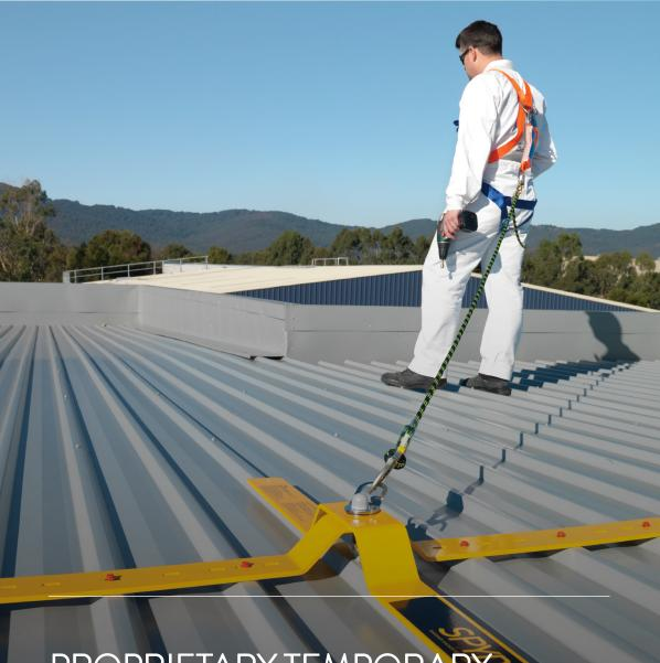
PROPRIETARY TEMPORARY ANCHOR SYSTEM FOR SAFE WORK AT HEIGHT
